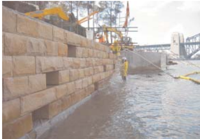
Final stages of rebuilding the seawall at McMahon's Point
