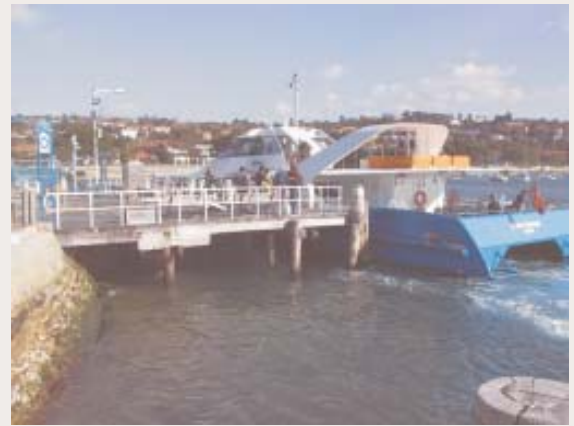
Wharf and Seawall at Rose Bay
