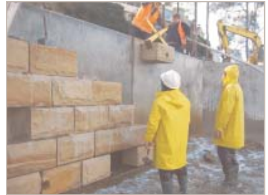
Building the seawall at McMahon's Point
