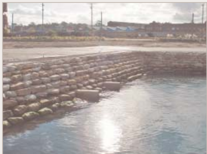
New seawall at White Bay
