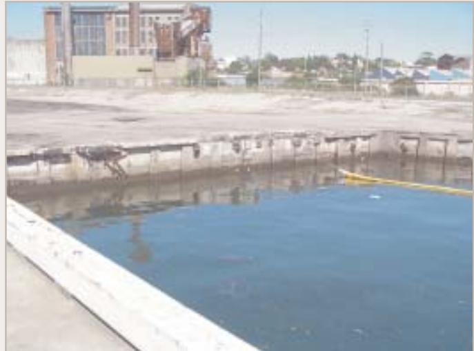
Old seawall, to be demolished (photo courtesy of Sydney Ports Authority)
