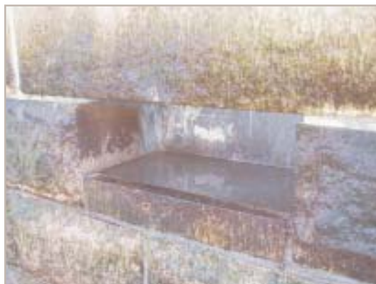
A pool embedded into the face of the new seawall
